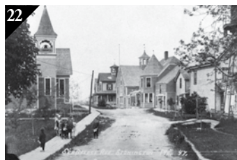
22 METHODIST CHURCH 10 SEABREEZE AVENUE Built in 1893, it has extensive tin work on the walls and ceiling. In 1915 Rev. Blake and a boy scout troop hand dug the basement creating a community room. At one time 200 children attended Sunday school.
