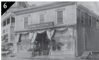
6 THE ISLAND AGENCY 26 MAIN STREET The building was built with a ground level store front and sided with cedar clapboards to add class to the clothing emporium, which later became the general store, Sturdee & Co.
