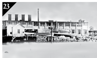
23 ISLE AU HAUT BOAT COMPANY 27 SEABREEZE AVENUE In the early 1900's, it was the Eastern Steamship Lines ferry terminal. Later, the North Lubec Sardine Canning Factory was built. It produced up to 100,000 cases a year until closing in 1992. Now the Isle au Haut Boat Services .
