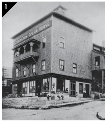
1 STONINGTON OPERA HOUSE 1 OPERA HOUSE LANE Russ's Music Hall , seating 900, was built in 1886. Renamed the Opera House in 1899, the building burned in 1910 but was rebuilt in 1912 with 256 seats. Entertainment included plays, silent movies, vaudeville, basketball games, dances and roller skating. Reopened in 1999 as Opera House Arts .
