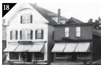
18 68 MAIN ST. (GWATSON GALLERY) Built as a large department store in the late 1800's it sold a full range of clothing and accessories on two floors!
