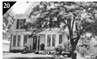
20 OCEANVIEW HOUSE 3 SEABREEZE AVENUE This 1883 building once had it's own windmill and water tank. The Lion's Club, who were instrumental in getting the bridge built, met here.
