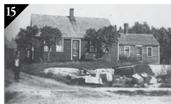
15 BOYCE'S MOTEL 44 MAIN STREET This early 19th century block frame house was a grocery store before the family built Boyce's Motel in front of the old house.
