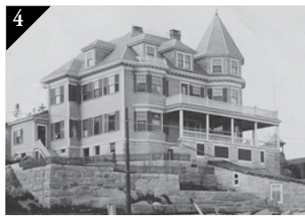
4 DR. NOYES HOUSE 39 MAIN STREET Built using granite quarried from the site in 1906. His patients joked, "Hope you're not too sick for the climb". Dr. Noyes had the first x-ray machine in Maine, 10 years after it was invented. Burnt in 1981, but rebuilt in 1986 on the same foundation.
