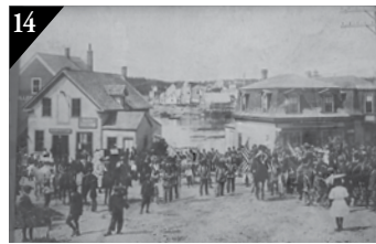
14 PENOBSCOT BAY PRESS 69 MAIN STREET In the 1880's, a patent medicine shop run by E.L. Frink, selling homemade cures. Later, Jim Stinson's Auto Repair and Stonington's first new car dealership. The westerly building was a stable, and quarry owner Job Goss's office.
