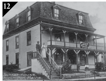
12 AMERICAN LEGION HALL 40 MAIN STREET Originally called Sunset House . The first floor was a bakery and lunchroom. Upstairs was a hall for the Knights of Pythias & Pythiaon, whose motto was "Honor, Loyalty, Freindship".
