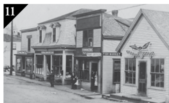
11 INN ON THE HARBOR 45 MAIN STREET An early version of a strip mall; including the first telephone office, a fish market, barbershop, post office, grocery, meeting hall and dentist office. The left hand building was brought in by barge.
